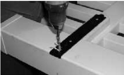
Using a 5/16" drill bit drill three perpendicular holes at least half way through the thickness of the gate.
